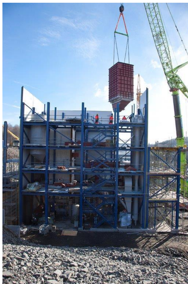
Image: Rottneros Mill's new bio-fuel boiler during construction
